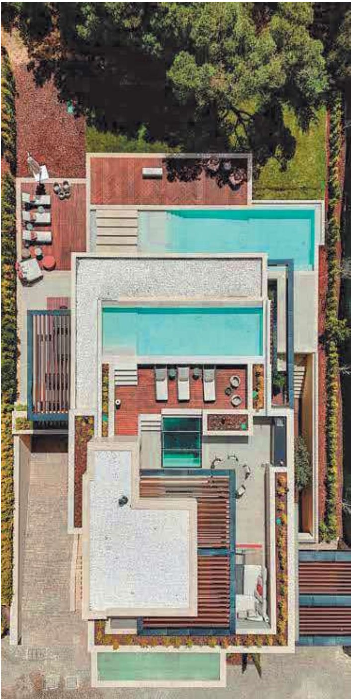
Above; Horizon Residence - Show Unit
