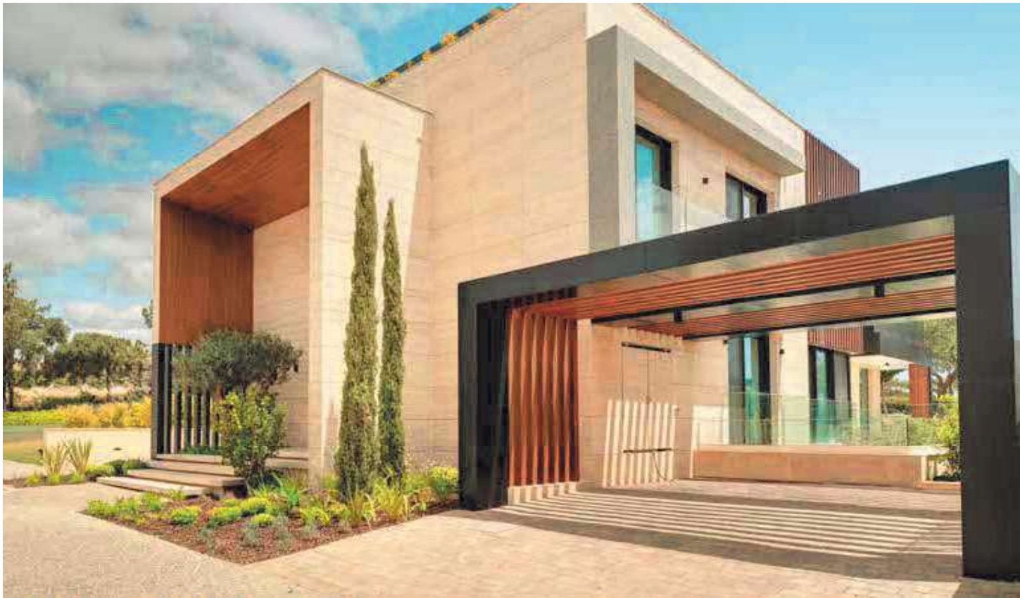
Above; Horizon Residence Show Unit
