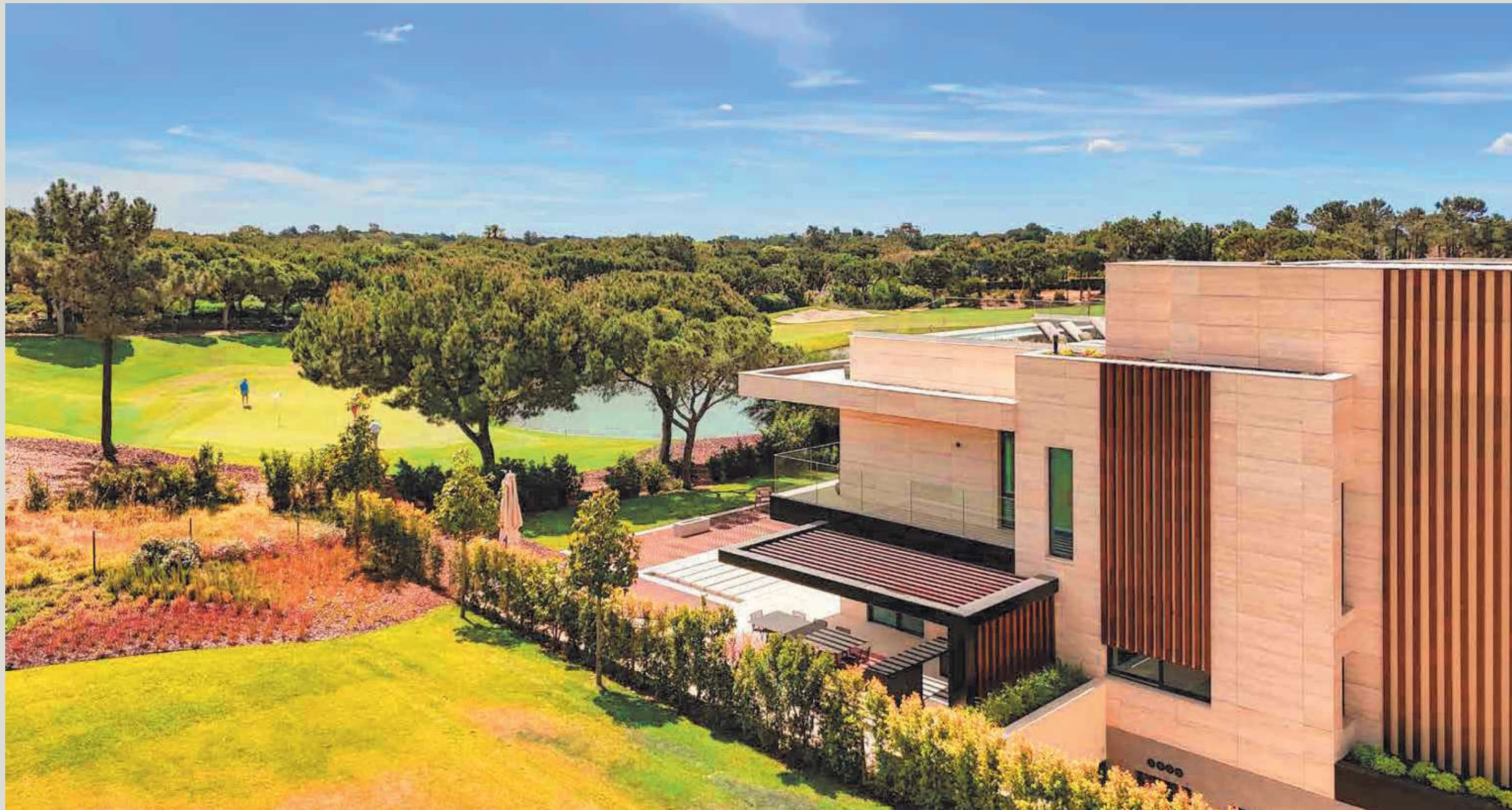
Above; Horizon Residence - Show Unit
